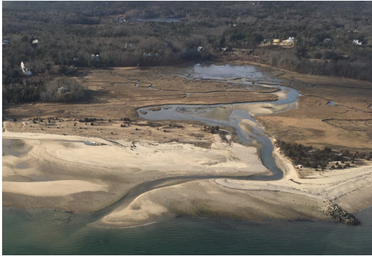
The diverted inlet prior to maintenance
