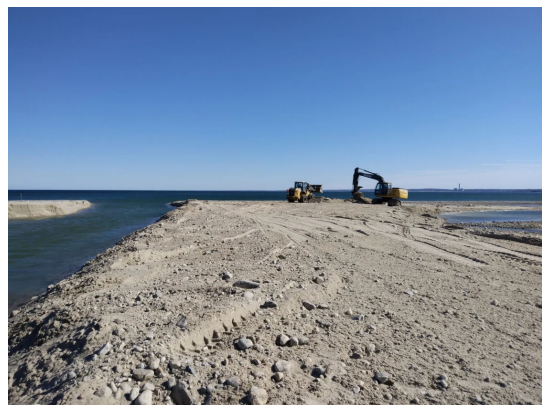
The inlet is restored to its most efficient path for tidal flushing. Photo courtesy of Eric Cody.
