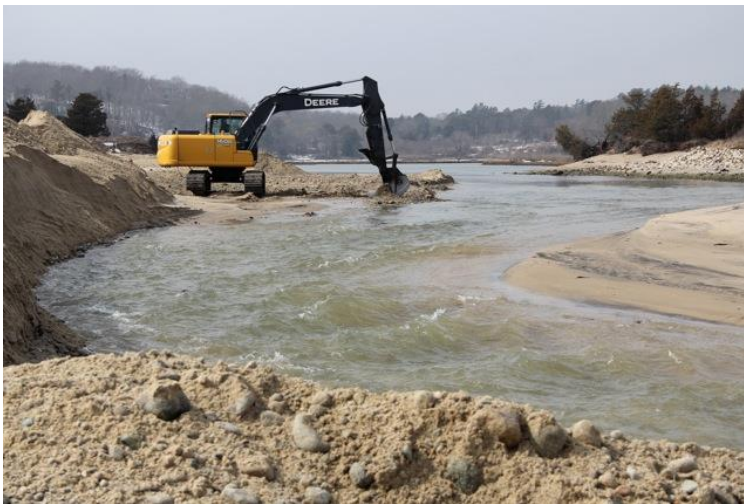
Channel Maintenance in March 2015
