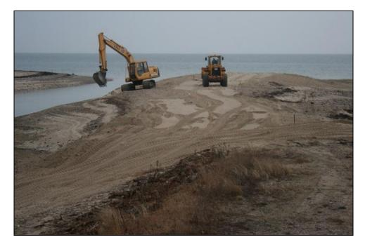
Final grading of the channel berm after closing the breach.
