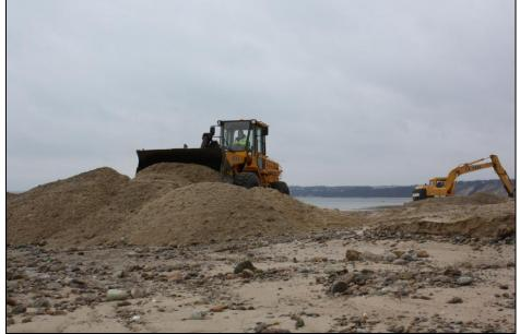
Richmond and Sons repair and rebuild the channel berm where it had been breached.
